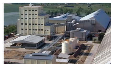
Bangladesh Chemical Industries Corp Chittagong Urea Fertiliser plant
