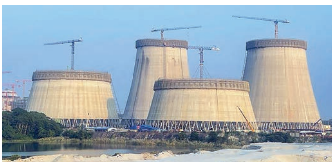
Photo right ● ROOPPUR NUCLEAR PLANT
