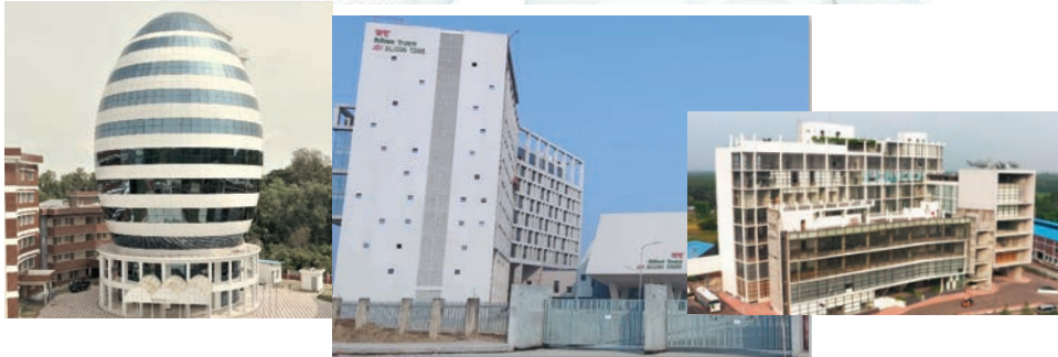
Operational ICT facilities in Bangladesh (Above row from left): Sheikh Kamal IT Business Incubator at Chittagong University of Engineering and Technology; Joy Silicon Tower in Bangabandhu Sheikh Mujib Hi Tech Park in Rajshahi and Solaris Building in Kaliakoir
