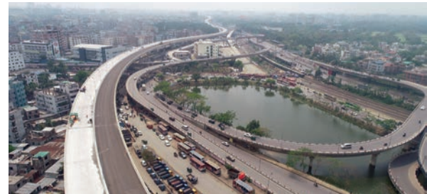
● DHAKA ELEVATED EXPRESSWAY: The already opened Airport-Banani section (Photo: Bangladesh Bridge Authority)
