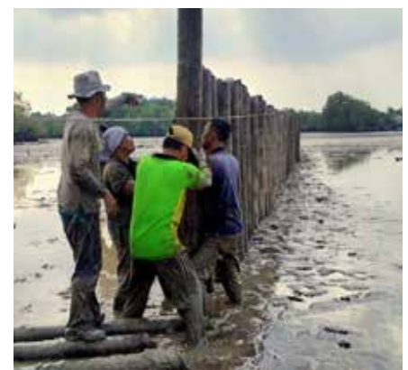
The local community constructing the wave breaker from Nibong trunks from the village to protect the planted mangrove in Buruk Bakul village.
