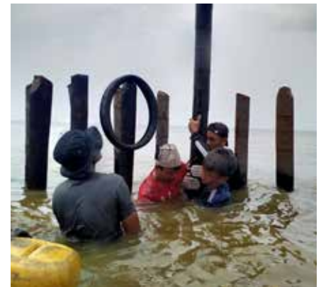
Buruk Bakul Village after the installation of a nature-based solution, 200-meter-long wave breaker made from Nibong palm trunks, to reduce wave energy and prevent coastal erosion.
